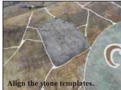
Engrave around the perimeter of the template. Nest another stone template next to the cut just made and engrave around it.
