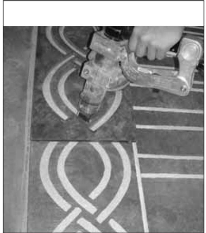
**Tilt the Shark each way to cut along the edges of the template.**
