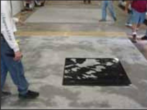
When using a four piece template set it is helpful to start by marking a cross hair in the center of the slab.
