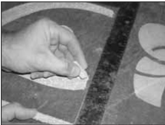
Layout the areas with a pencil or chalk and use the wasp to remove the concrete.
