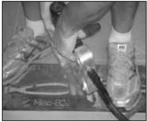
Hold template in place by either standing on it, or by anchoring it with concrete screws.
