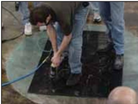
When cutting next to the template edges, slightly angle the impactors toward the side of the template. This gives crisp edges on the design.
