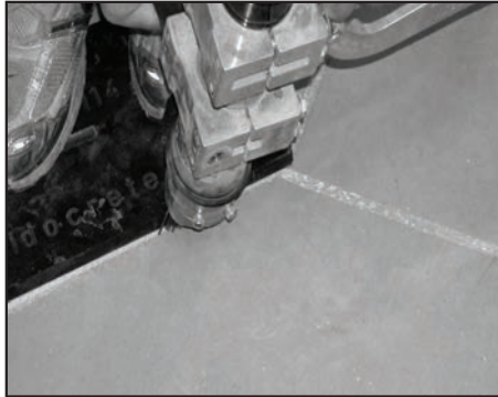
Align template slot marks with snapped chalk lines.
