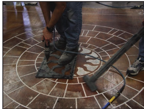
Rotate template 180 degrees, align and engrave second half
