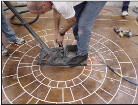
Rotate template 180 degrees, align and engrave second half
